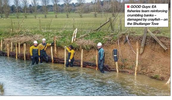
bundle reinforcing to bolster collapsing banks, banks undermined by burrowing red signal crayfish.
